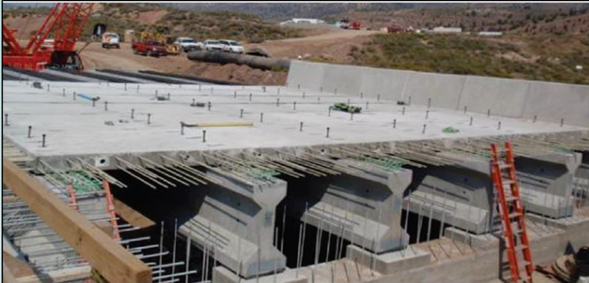
Application of FRP as internal reinforcement, Emaa Park Bridge deck panel with GFRP reinforcing bars (ACI 440.1R-15)
